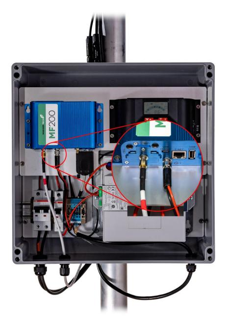
Step 14 - Switch on / plug in all circuit breakers inside the enclosure.
