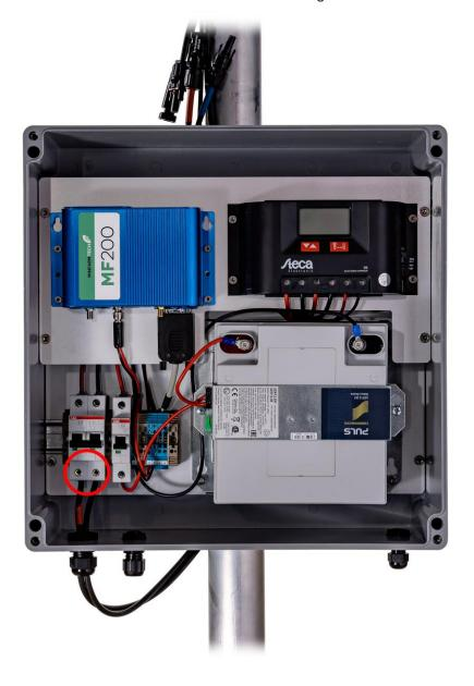
Step 11 - Connect both sides of the solar panel.
